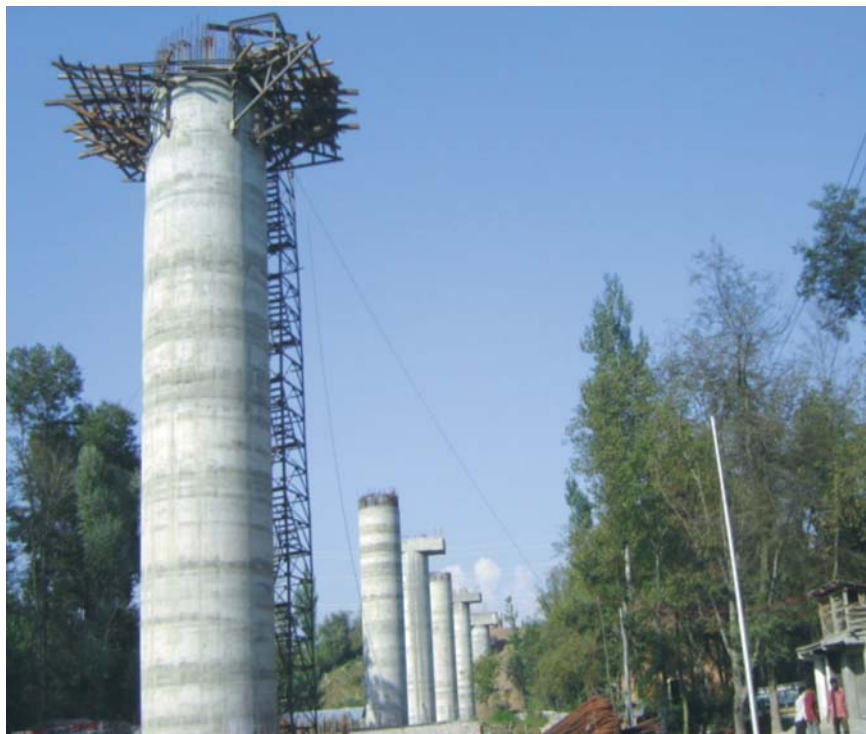
Construction of Veith bridge (Jammu-Udhampur line) in progress.
