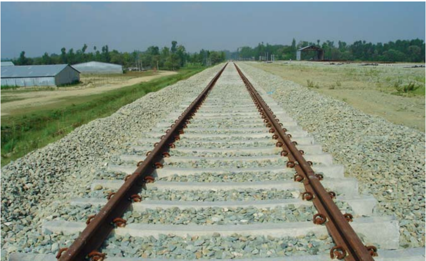
Completed track on a section of Jammu-Udhampur rail line.
