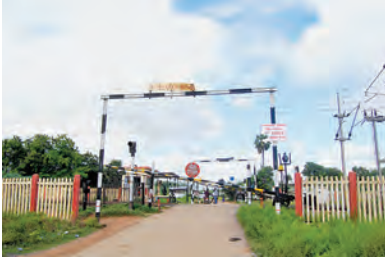
Train Actuated Warning Device (TAWD) at UMLCs, SR
