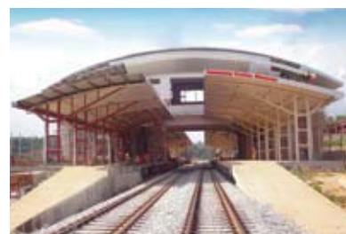
Construction work of Senewang Railway Station at Malaysia undertaken by IRCON.
