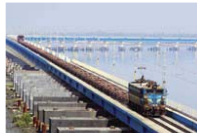
Railway bridge connecting Idapalli and Vallarpadam, RVNL.
