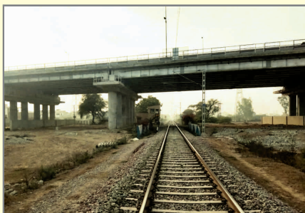
Road over bridge provided in lieu of level crossing Nos. 47-A in Bathinda - Sri Ganganagar section
