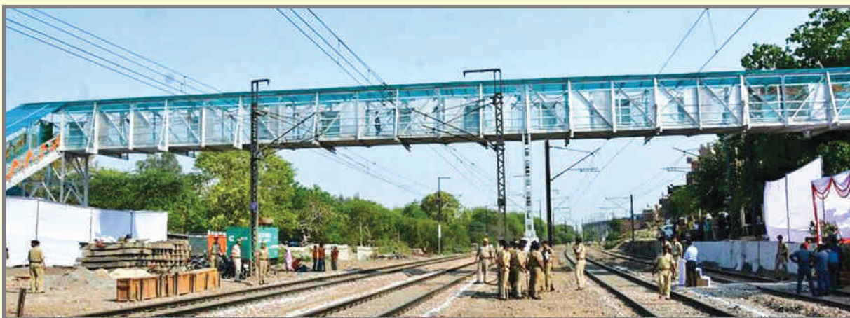
Inauguration of newly constructed Foot Over Bridge (FOB) at Harkesh Nagar, New Delhi by Hon'ble Former Minister of State for Railways, Shri Manoj Sinha and MP, Shri Ramesh Bidhuri
