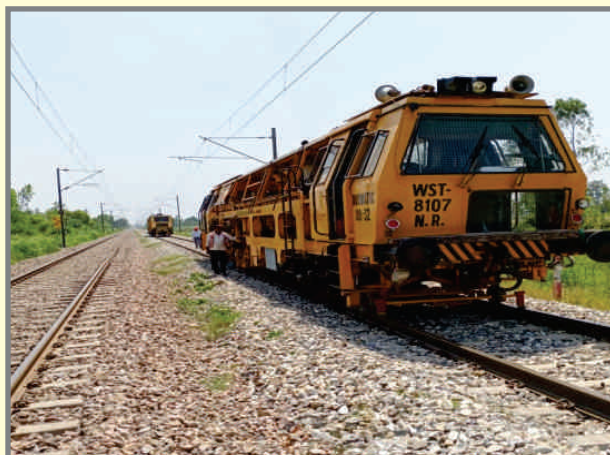
Use of state-of-art UNIMAT and Tamping Machines for renovation of tracks
