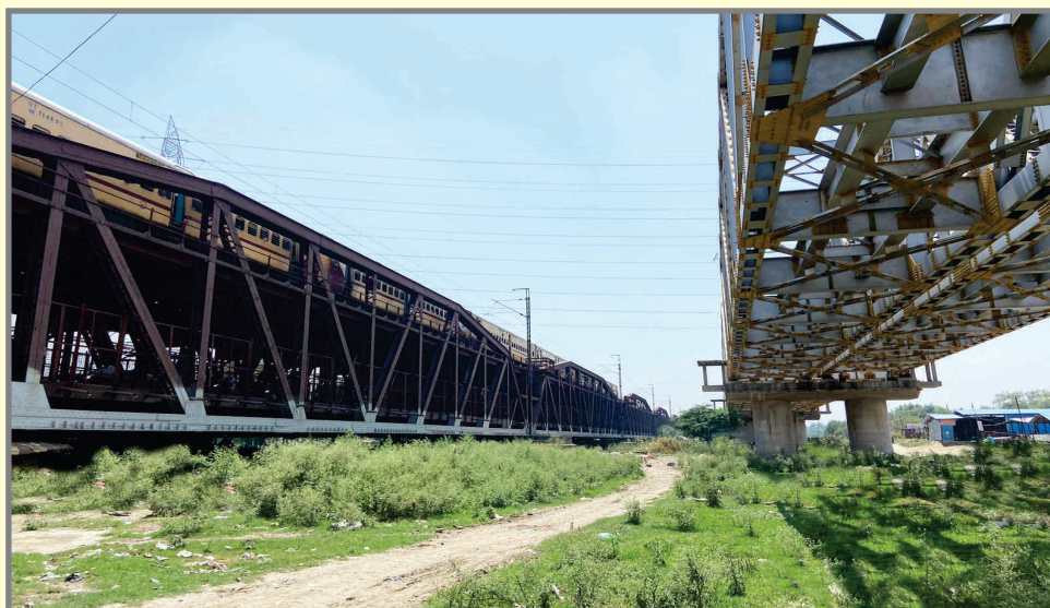
New Bridge across Yamuna being constructed besides Lohe Ka Pul
