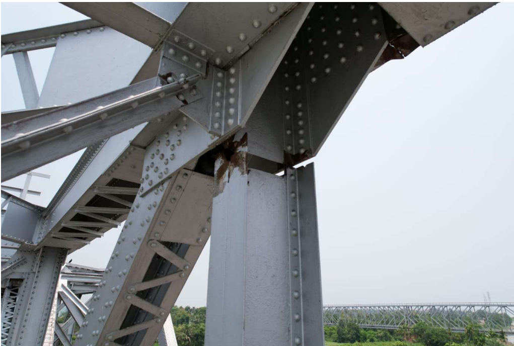
DISTORTION IN THE TOP CHORD MEMBER
