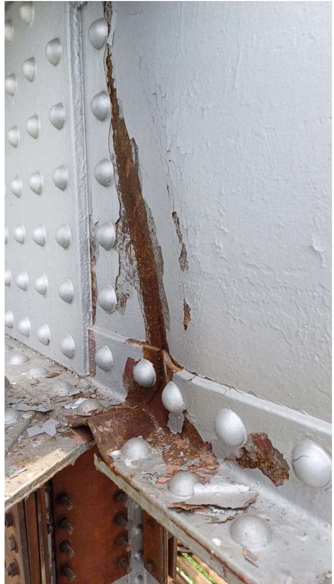
WARPING IN TOP CHORD WEB/ANGLE
