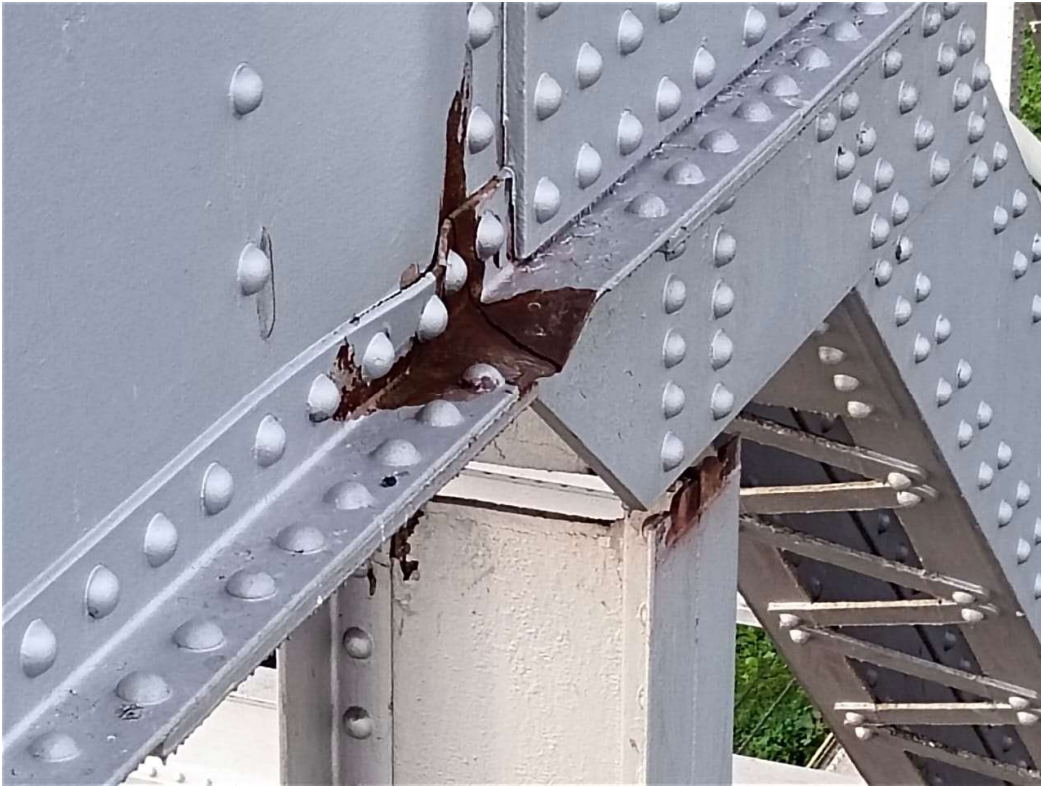
DISTORTION IN THE TOP CHORD MEMBER
