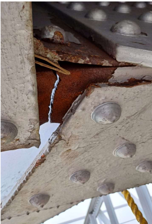
GAP OF 65mm OCCURRED IN THE VERTICAL
