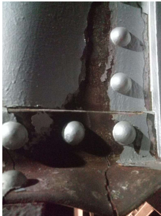
CRACKS AT JOINT "U1"
