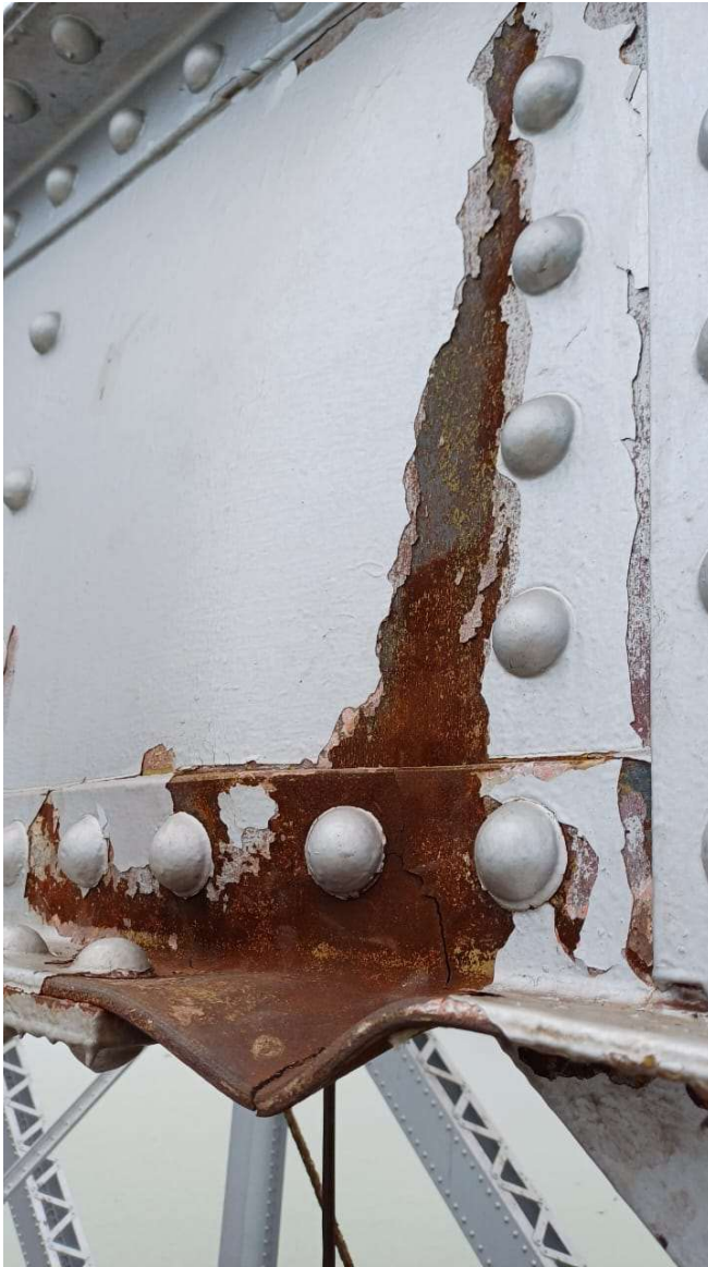
WARPING IN TOP CHORD WEB/ANGLE
