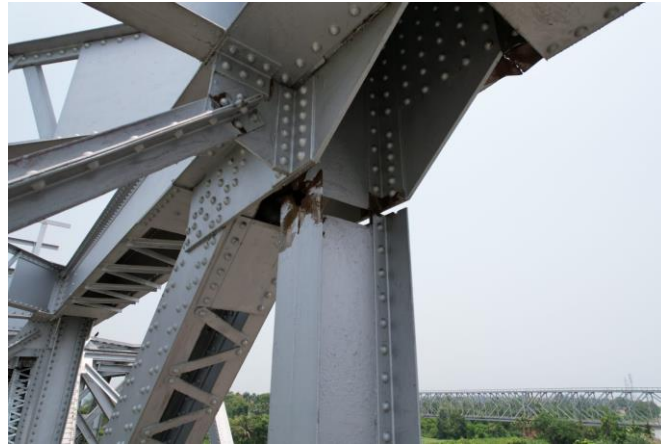
Fig.1: Full crack near U1 Node in the line of the last rivet (from Top) in Vertical & Gusset Connection.
