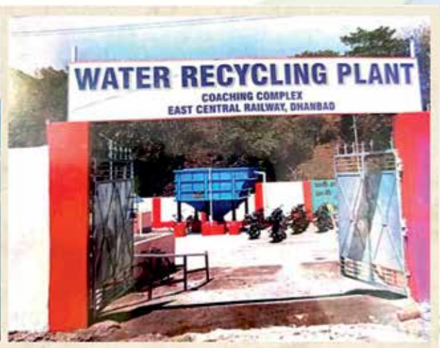
WRP commissioned at Coaching Complex Dhanbad
