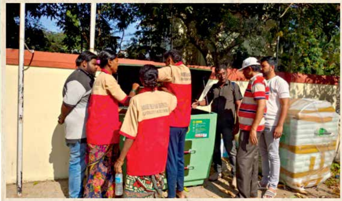
Installation of composter boxes at Rail Nagar Colony
