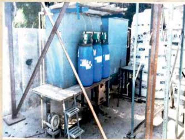
ETP of capacity 05 KLD installed at Bikaner Workshop during the year 2023-24
