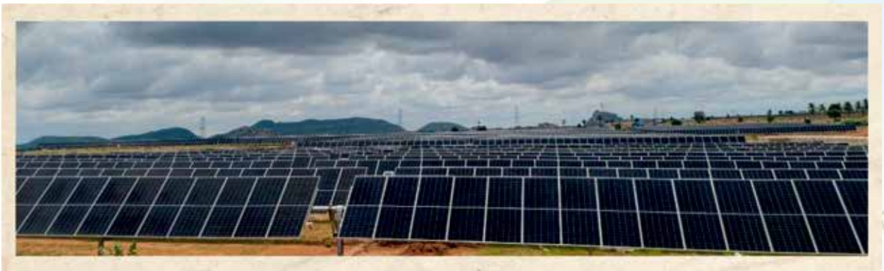
Solar plant by IRCON in Pavagada, Karnataka
