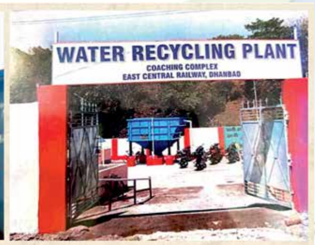
WRP commissioned at Coaching Complex Dhanbad
