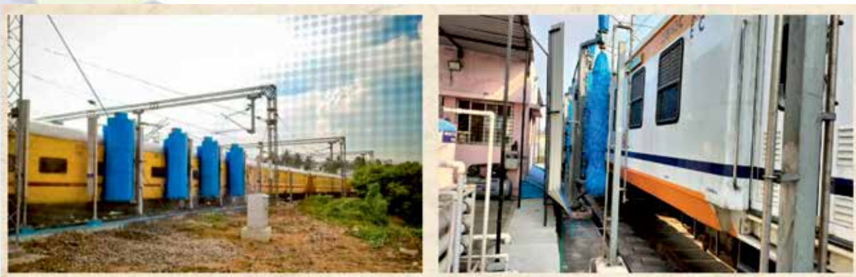
ACWP at Mysuru shed
