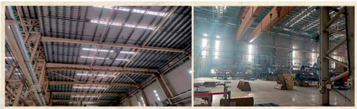
Diesel Locomotive factory, Marhowra
