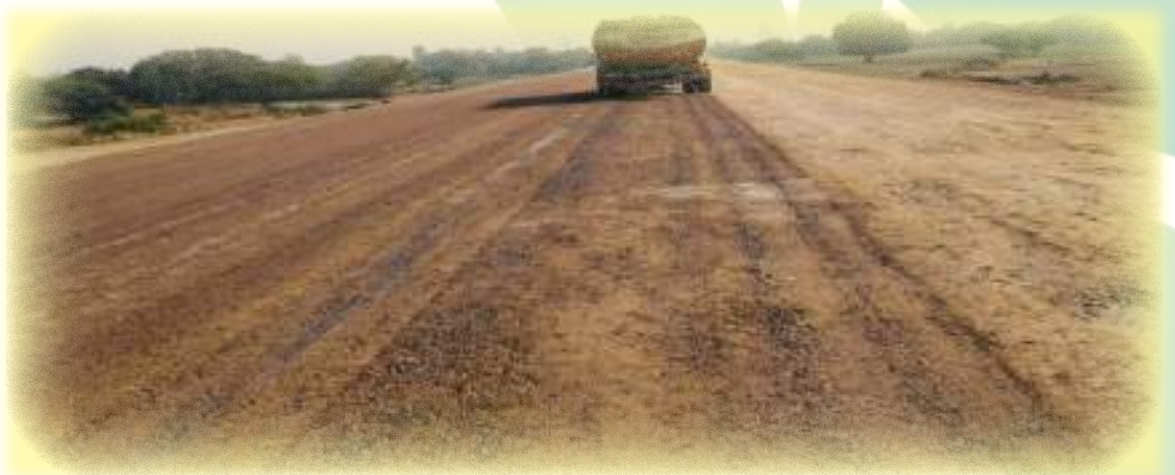
Fly ash utilization in formation of embankment at waterlogged area
