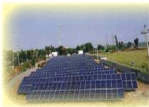
Solar Plant Feeding into Traction Sub-Station Installed at Diwana
