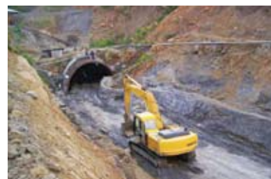
Tunnel construction work – Lumding-Silchar gauge conversion (National Project), Northeast Frontier Railway.
