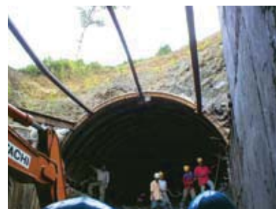
Tunnel construction work – Lumding-Silchar gauge conversion (National Project), Northeast Frontier Railway.
