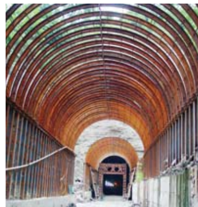
Tunnel construction work – Lumding-Silchar gauge conversion (National Project), Northeast Frontier Railway.
