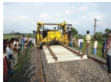
Gauge conversion work at Katihar - Mukuria section, Northeast Frontier Railway.
